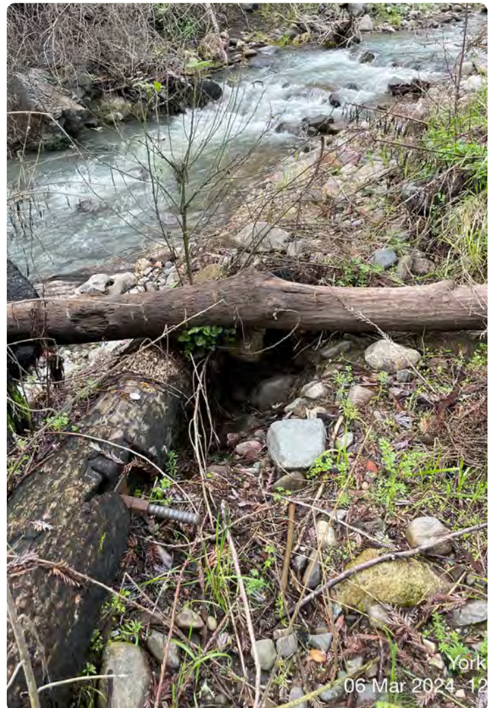
Log structure at WRA's York Creek project supporting ecological function and impounding sediment.
