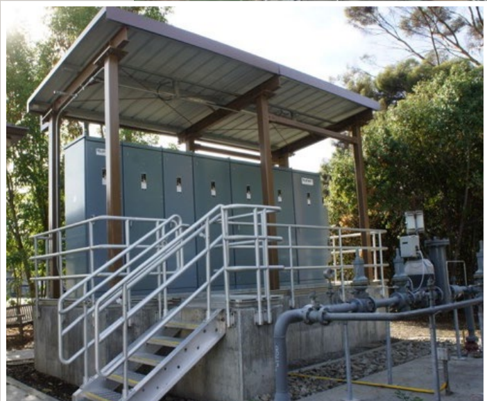
Elevated power distribution equipment
