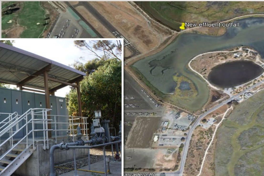
Elevated power distribution equipment
