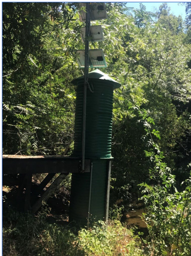
Figure 5-3: San Francisquito Creek at Stanford Gage Stilling Well
