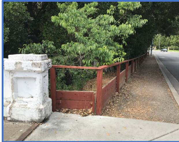
Figure 2. Temporary Wooden Wall, University and Woodland Avenues, East Palo Alto
