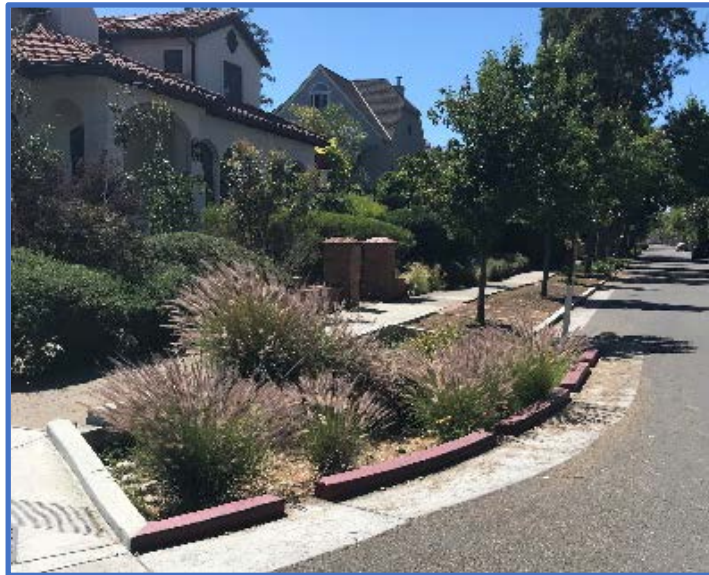
Figure 6. Bioretention Basin Example, Southgate Neighborhood, Palo Alto
