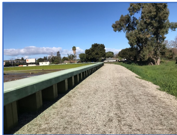
Figure 5 Example of sheet pile installed downstream
