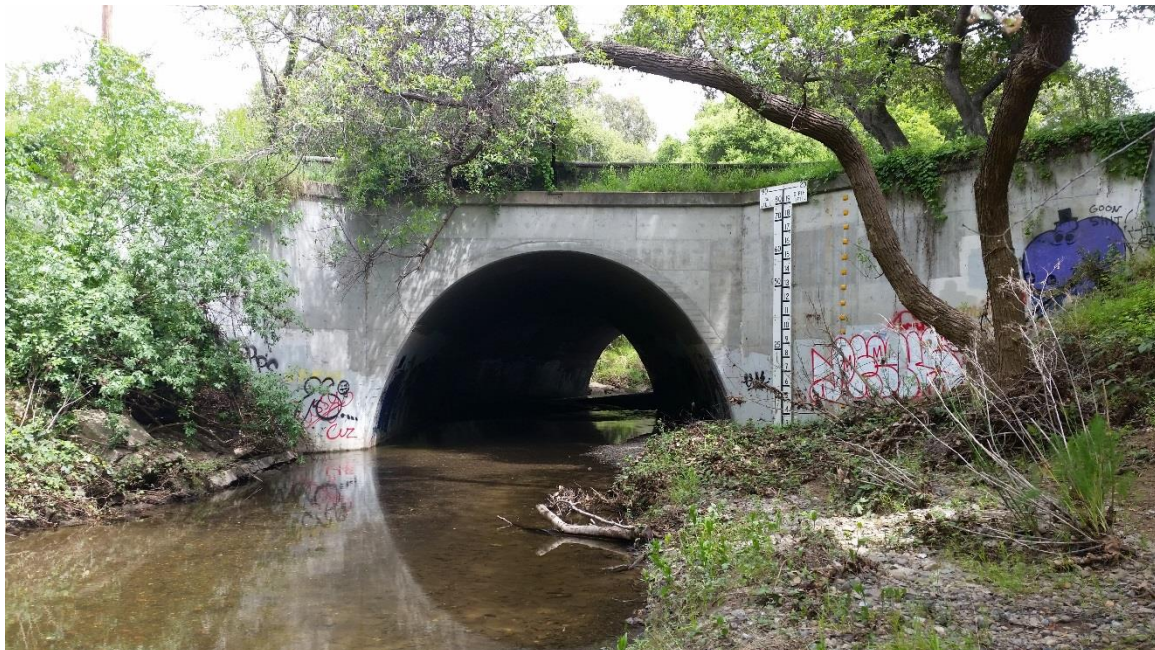
Overview of the north side of the Pope-Chaucer Bridge, view southwest
