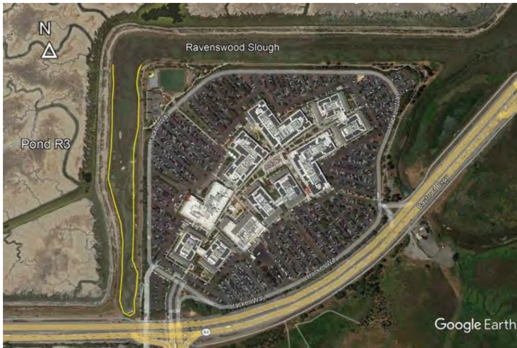
Ravenswood Slough shoreline with base of 84-foot levee extending west from Hacker Way, showing increased convergence of the shorelines.
