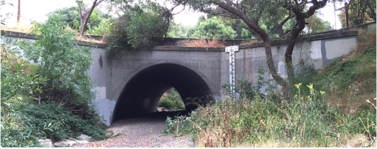
Existing Pope-Chaucer Bridge
